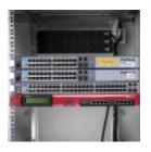
Level 3 EMP cabinets are equipped with shielded connectors for both power and fibre optic cables. These in conjunction with the Faraday properties of the cabinet ensures that the stored equipment and information is
